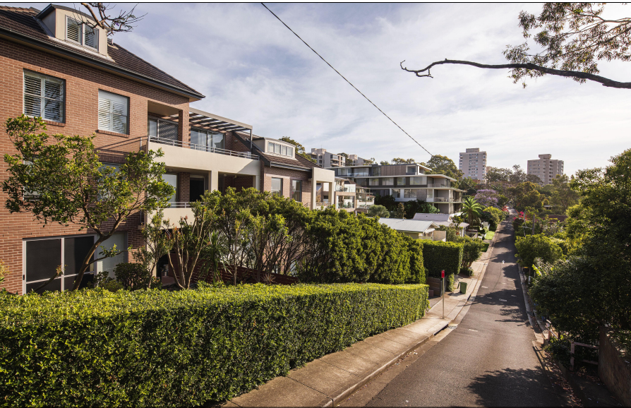
GERARD LANE THROUGH TO BENELONG ROAD
