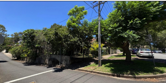
STREET TREE AND POWER POLE TO CORNER OF BENELONG RD & GERARD LANE
