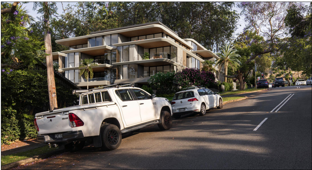
BENELONG ROAD THROUGH TO GERARD STREET
