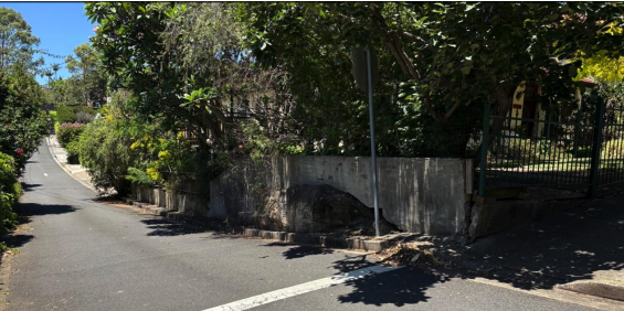
No. 118 BENELONG RD RETAINING WALL ON GERARD LANE
