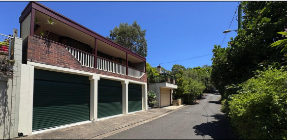
No 72 GERARD ST DRIVEWAY VIEWED FROM GERARD LANE
